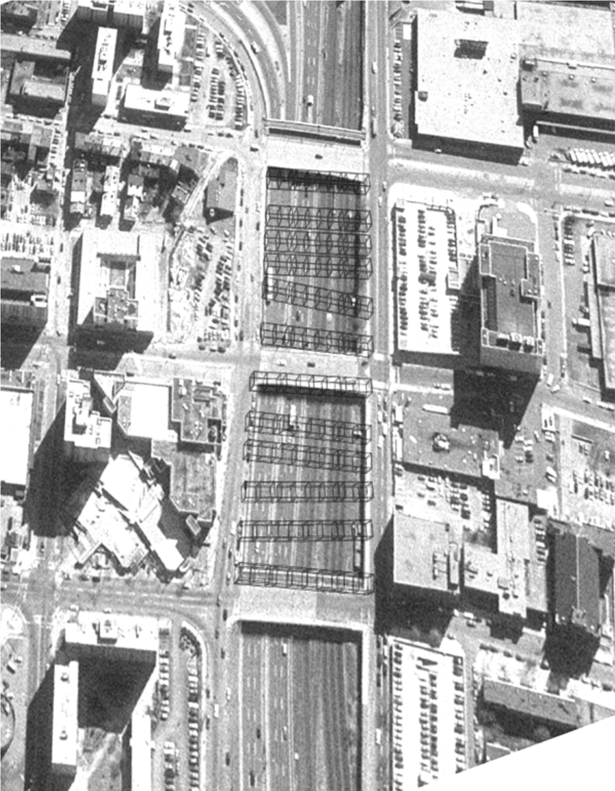
Fig. 10 Vierendeel trusses over the Mass Pike
